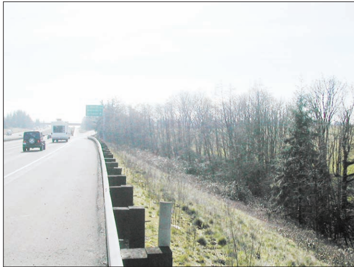
View from I-5 looking south onto the La Center Interchange Site.
