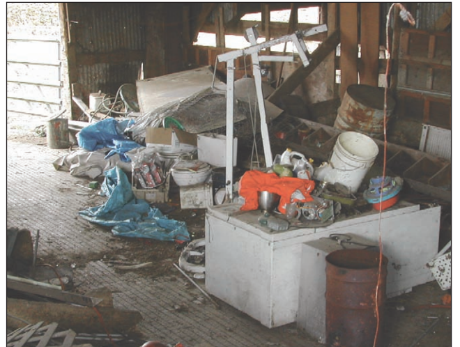
PHOTO 9: More non-hazardous debris located in one of the barn areas.
